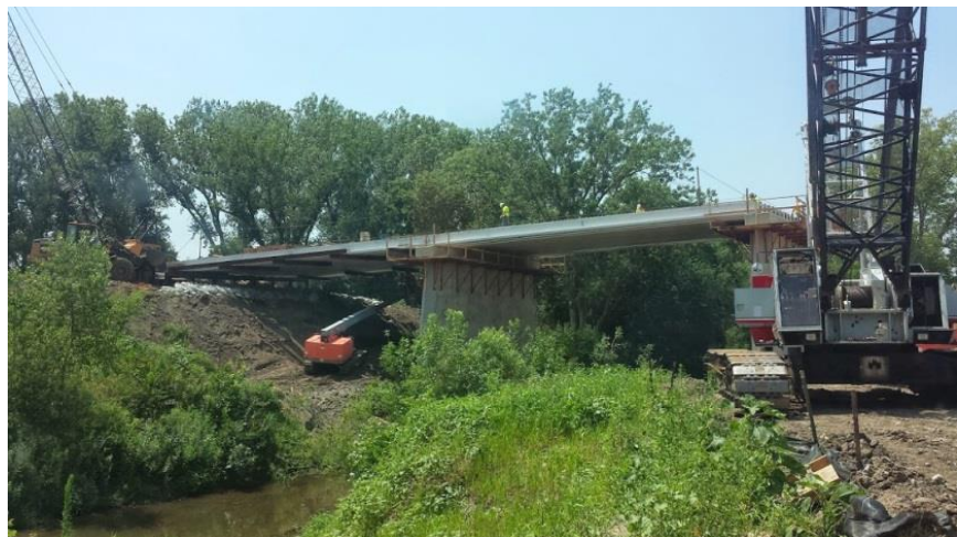
Figure 2: South side of the SW 40 th Street viaduct
