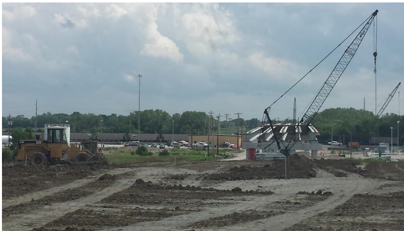
Figure 1: North side of the SW 40 th Street viaduct project
