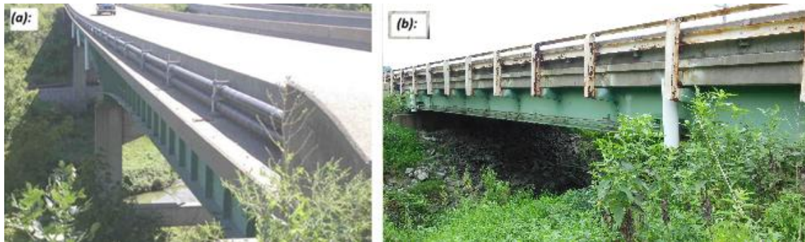
Figure (1). two bridge candidates which sensors mounted on, (a): three-span US20 Bridge in Dubuque FHWA #23850, (b): single span bridge IA-21 Hwy in Keokuk County FHWA #32600.
